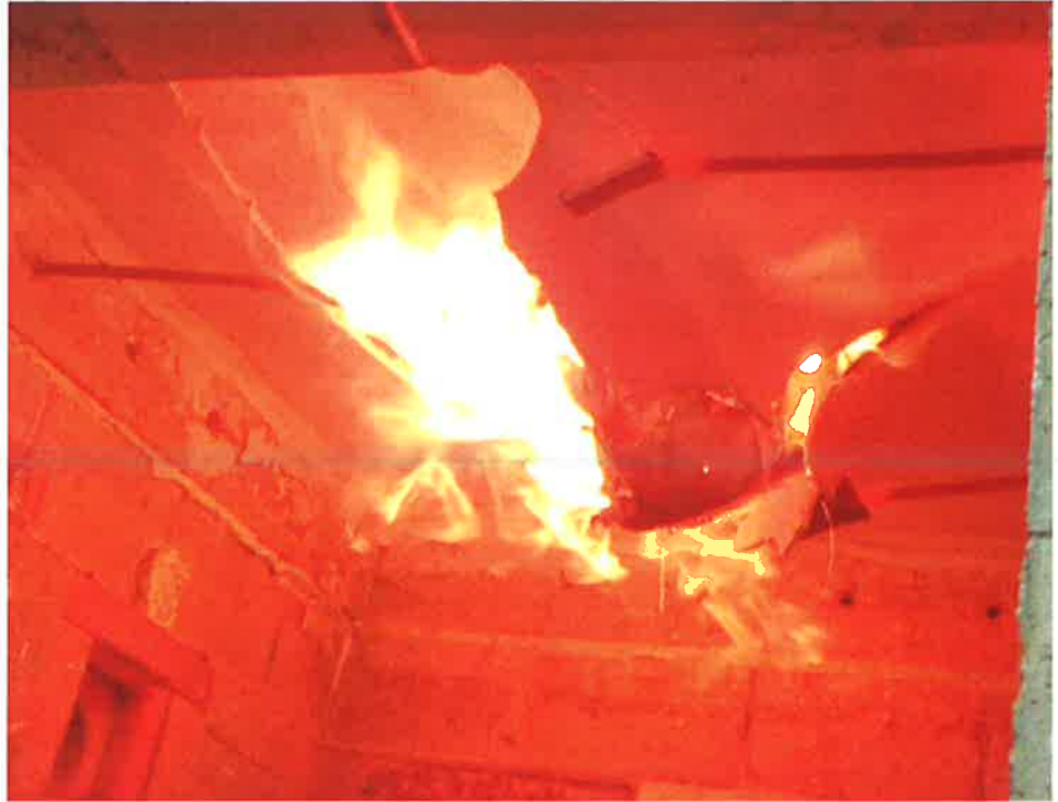
The exposed face of the ceiling immediately after the test
