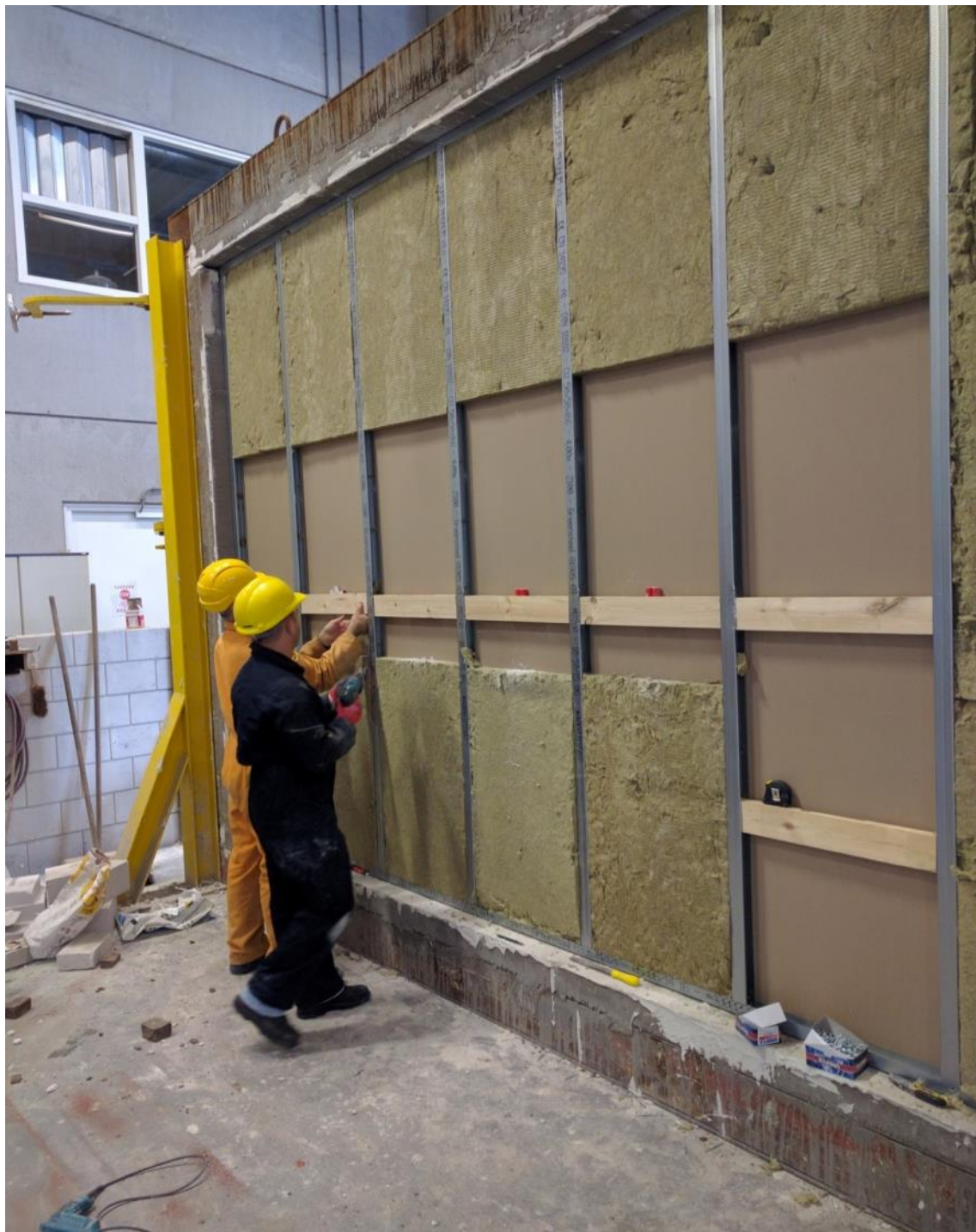
Photo 1 Timber installed for support of the hollow wall boxes
